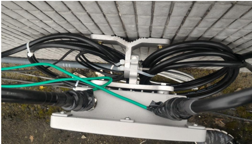
Figure 30 Lightning Protections and Grounding Equipment – Image 1
