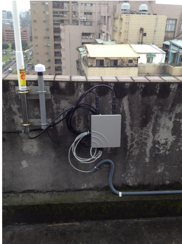
Figure 32 6 PVC cable protection hose
