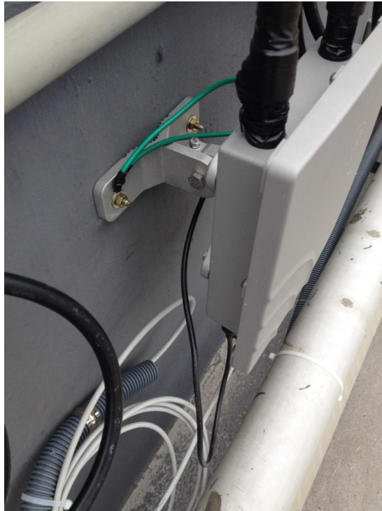
Figure 31 Lightning Protections and Grounding Equipment – Image 2
