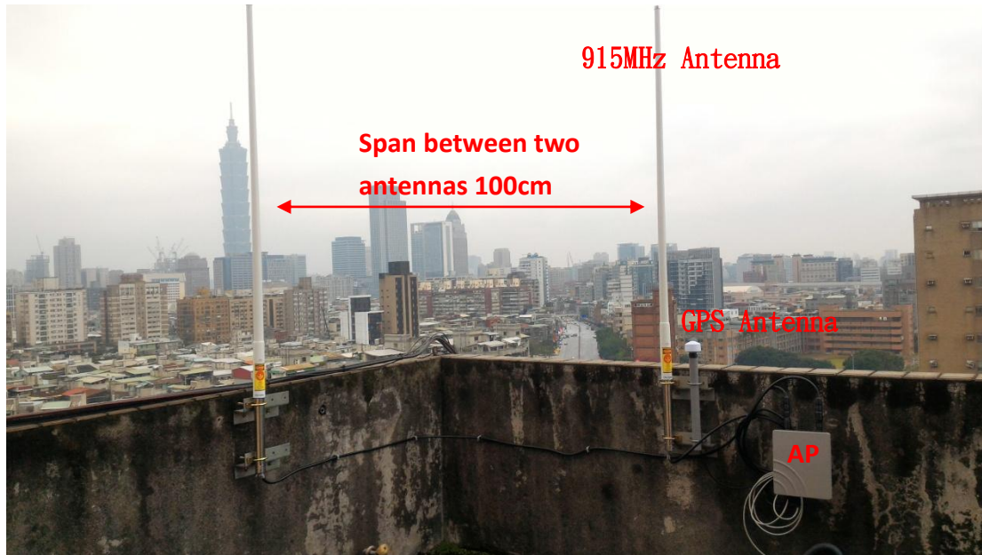
Figure 21 Actual View of a Wall-mount Installation
