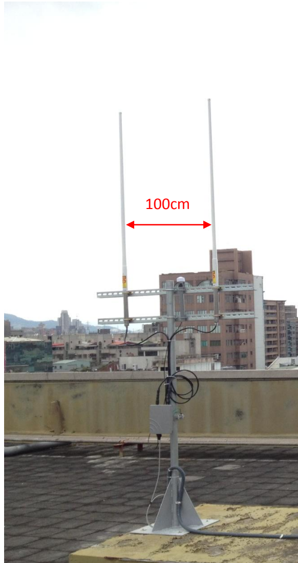
Figure 33 Actual View of a Base-mount Installation
