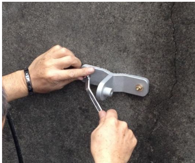
Figure 22 Wall-mount Installation – Image 1
